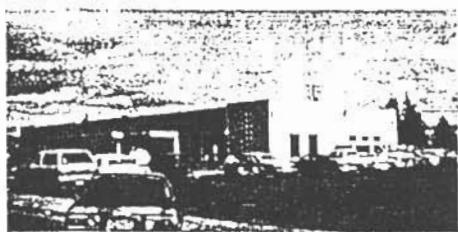
Fig. 5. Elk's Lodge No. 1613 served as central command post for the building inspection services.
