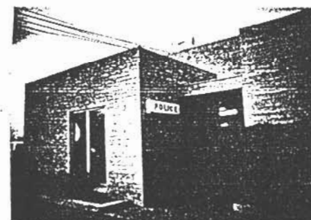
Fig. 14. Police headquarters — The reinforced concrete masonry survived without damage.
