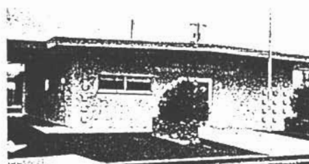
Fig. 13. Department of Motor Vehicles — No damage to the concrete masonry building.
