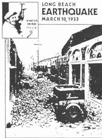
Fig. 2. Damage to unreinforced masonry buildings in the March 10, 1933, earthquake of Long Beach.
