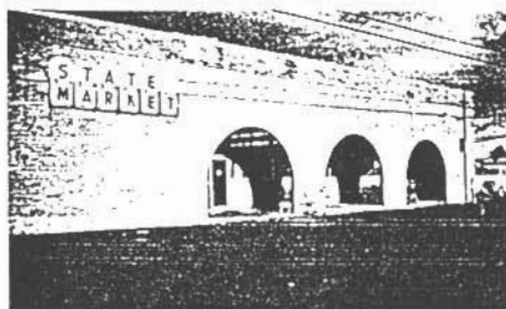
Fig. 11. State Market — reinforced masonry; no damage.
