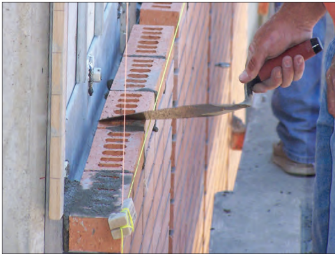
Figure 6 Masons laying to line
