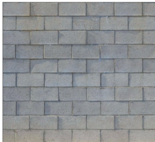
Figure 4 Improper evaluation of CMU wall with the sun shining directly overhead
