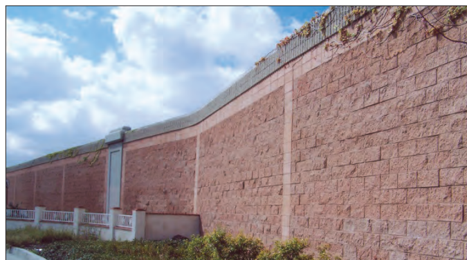
Figure 2 Split face or slumped concrete masonry units intentionally creating shadows and texture
