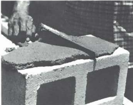
SPREADING mortar on masonry unit.
