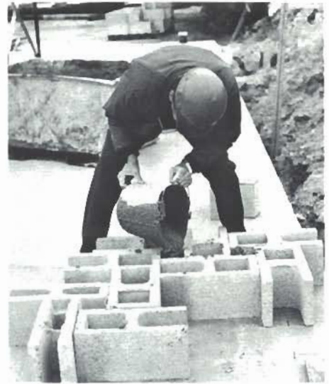
POURING grout into molds made of masonry units.
